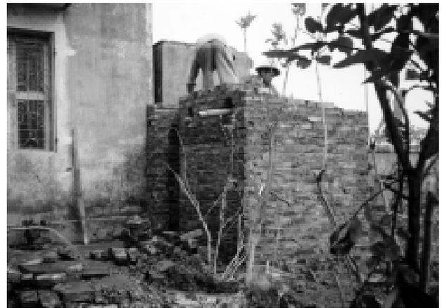
*Brick masons build the walls for new bathroom.*
